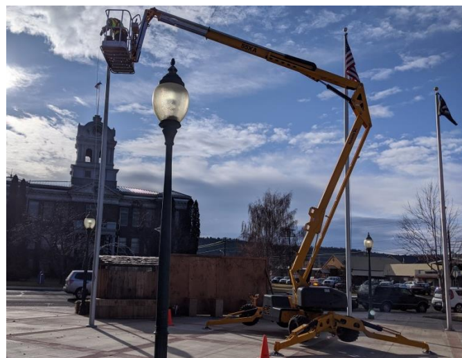
New flags being installed by IT in the plaza
