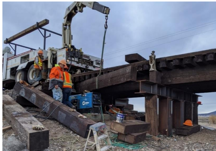
Railway bridge work done during the second quarter
