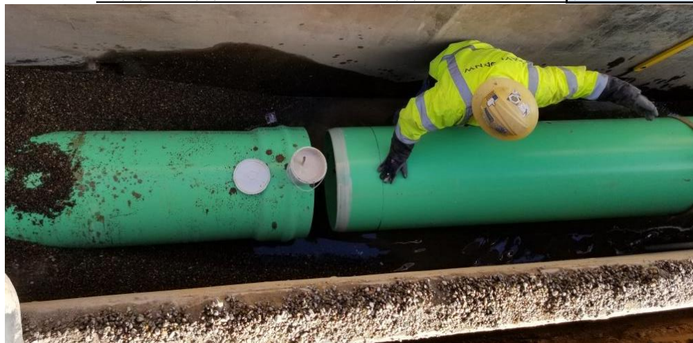
Sewer interceptor project at 10 th and Main Street
