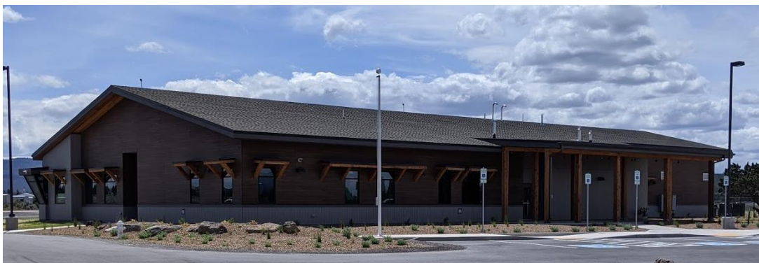
New USFS building at the Prineville Airport that was ready for occupancy during the fourth quarter.
