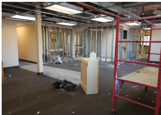
Demolition to the new Police building during the fourth quarter.
