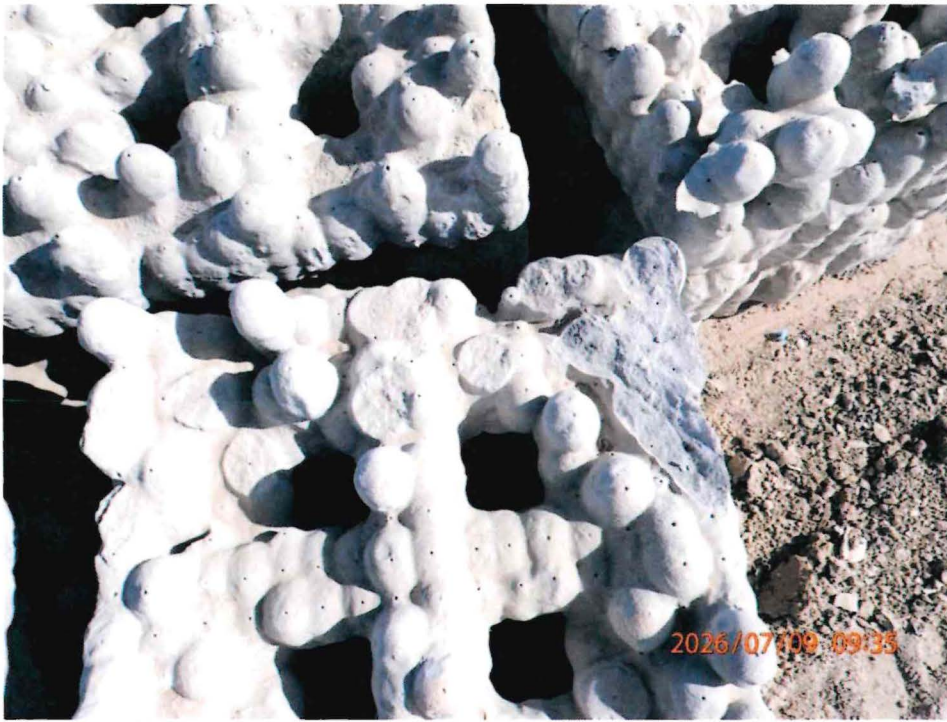
Figure 1. ARU with large fracture of lattice brush removed.
