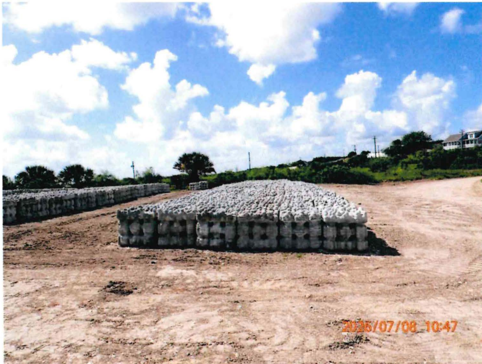
Figure 4. ARUs stockpiled at Borrow Site B.
