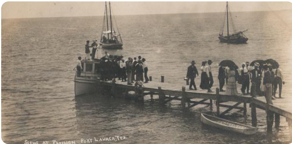
Figure 2: Historic Image, Scene at Pavilion, Port Lavaca, Texas
