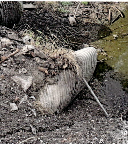
View of collapsed pipe on upstream side after clearing operations
