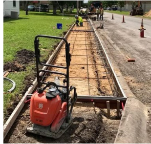
Sidewalk Installation on Bauer Street. Source: City of Port Lavaca
