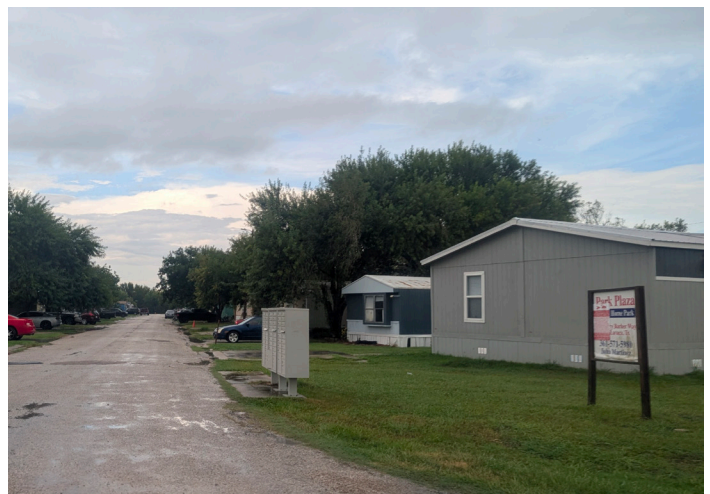
Manufactured homes at Park Plaza Mobile Home Park in Port Lavaca Source: Baxter and Woodman
