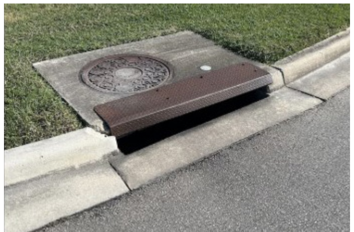
Stormdrain in San Antonio, TX Source: Joint Base San Antonio
