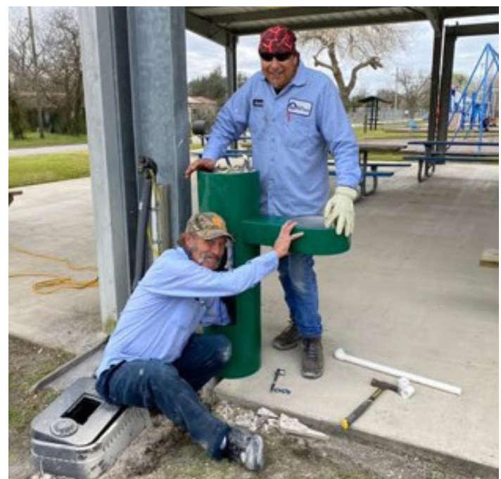
Staff install new drinking fountain at George Adams Park Source: City of Port Lavaca
