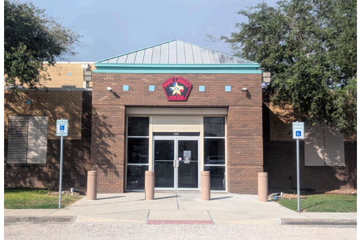
Port Lavaca Police Department Source: Baxter and Woodman
