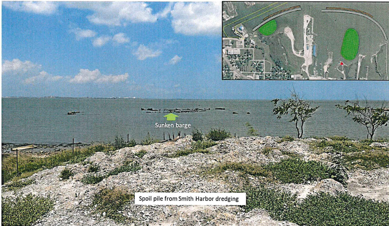
Figure 2. Spoil mound from recent dredging of Smith Harbor (foreground) and a sunken barge just offshore. There are no plans in the grant to remove the barge and should be considered when designing the marsh creation cells.
