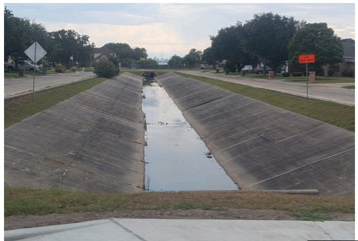
Drainage Ditch along La Salle Boulevard in Port Lavaca Source: Baxter and Woodman
