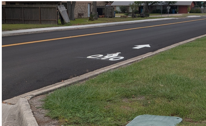
Bike lane on Smith Road in the process of being striped Source: City of Port Lavaca
