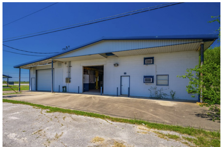
Port Lavaca Warehouse Source: Republic Commercial Land and Brokerage (placeholder)
