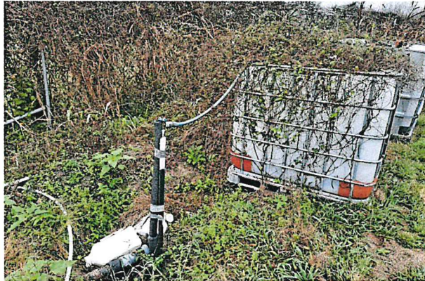
No. 5 Parcel 3 - Piping stick-up and totes
