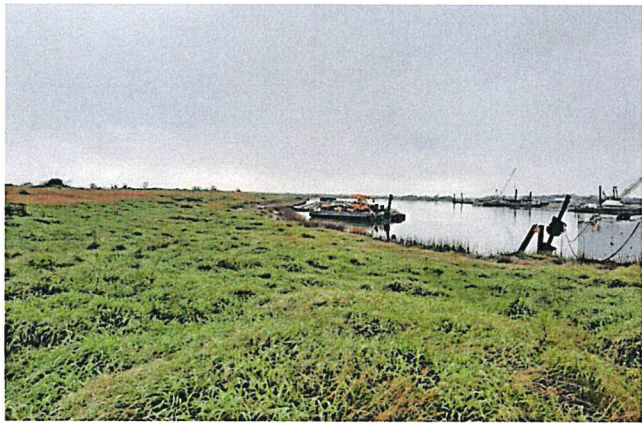
No. 9 Parcels 11 & 12 - Dredge pipe staging west of Parcel 12
