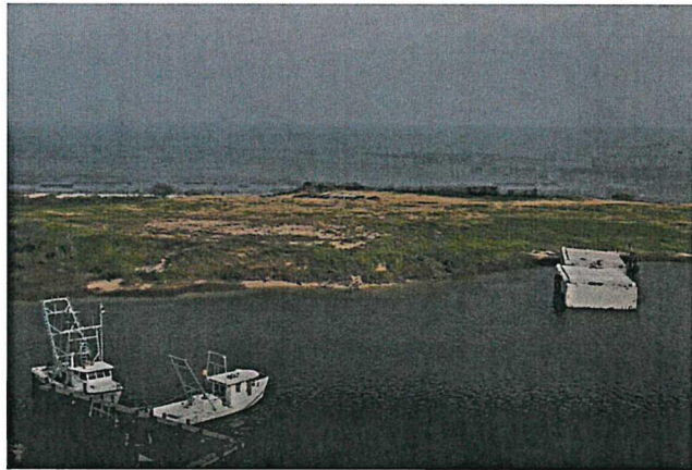
No. 12 Parcel 11 - drone photo (provided by CoPL), distressed area and piping
