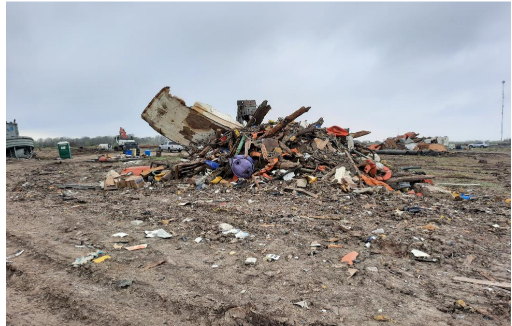
No. 4 Debris pile for disposal.
