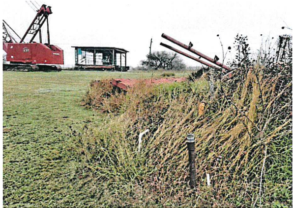
No. 6 Parcel 3 - Piping stick-up and debris pile
