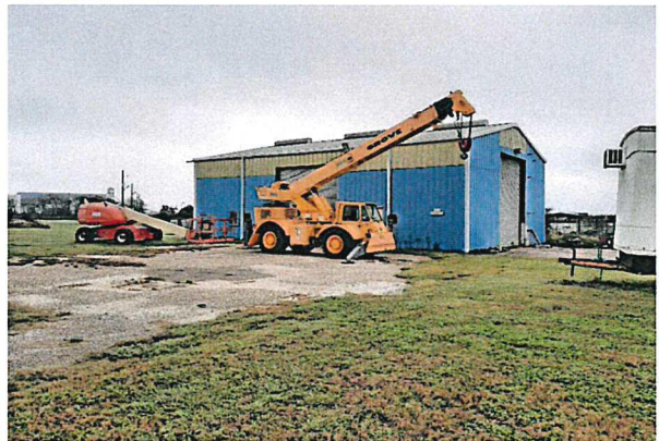
No. 4 Parcel 3 - Building, crane, manlift.
