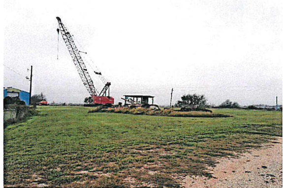
No. 2 Parcel 3 - Crane and floating dock debris.
