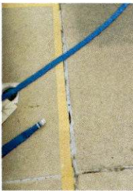
Photo 11 – Description: Skimmer Pic
