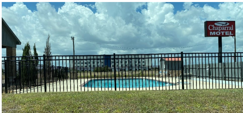
Aluminum fencing – similar to that around the pool at Chaparral (there is a 3 rd horizontal bar near the ground, hidden by the berm in this photo)
