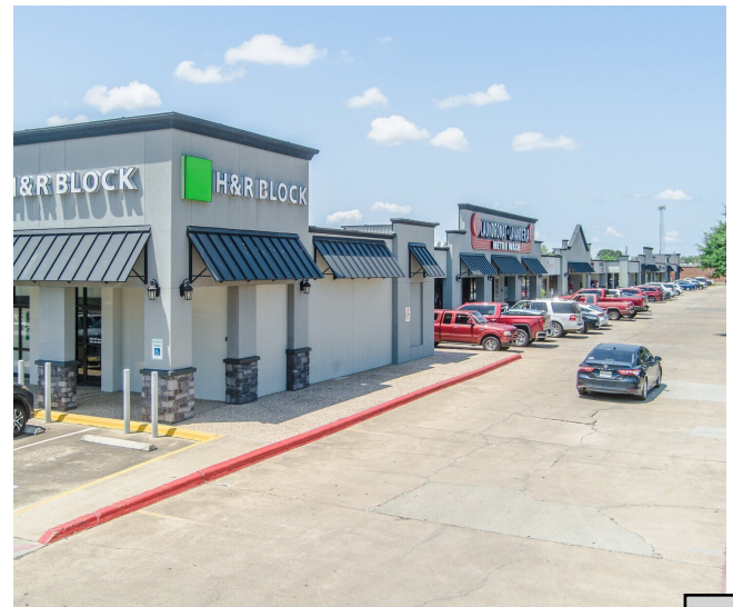
Red River Street auto-urban commercial property in Victoria, Texas Source: Belinda Realty
