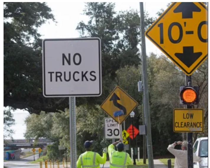
Installation of truck route signage alerting trucks of low clearance.
