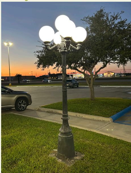
Pedestrian scale lighting and taller street lighting in Port Lavaca Source: Baxter & Woodman
