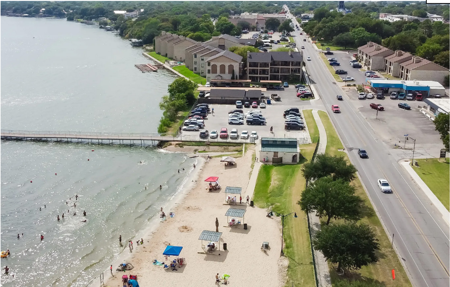
Granbury, Texas, has developed a 10 to 12-foot wide shared-use path following Business US-377 and their Brazos River waterfront connecting a public beach, their downtown, hotels, and the local conference center. Source: Visit Granbury
