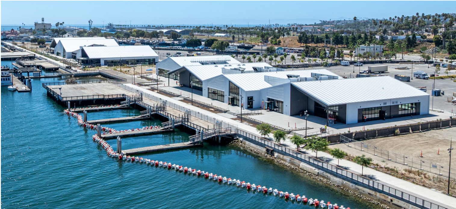
West Harbor revitalization project in San Pedro, California, pictured with newly constructed harbor buildings, landscaping, shoreline stabilization, and public access walkways and boat docks Source: CoStar News, Brannon Boswell
