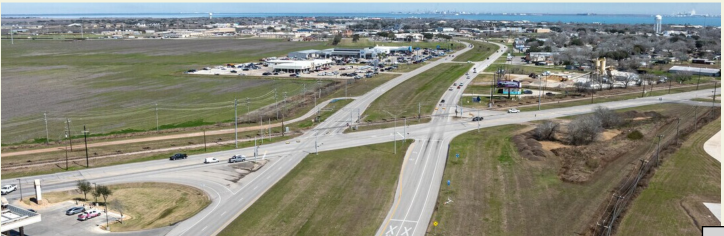
Aerial view of Port Lavaca from the SH 35 and US 87 Interchange Source: Homes.com
