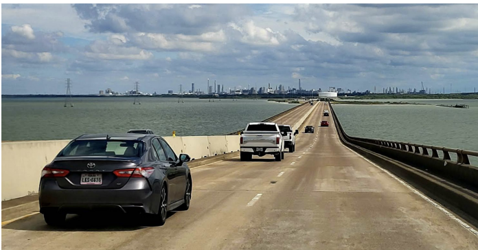
Port Lavaca Causeway heading towards Point Comfort
