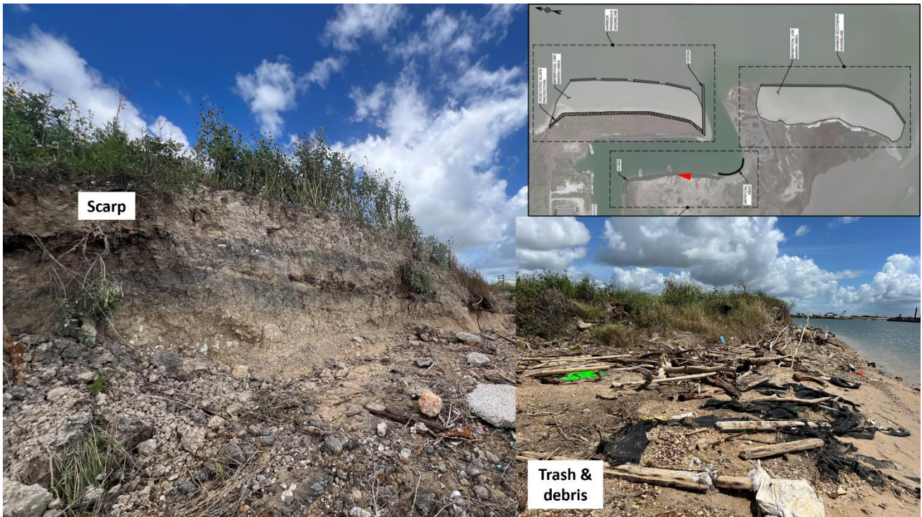
Figure 2. High scarps (estimated to be taller than 5 ft) and trash along the inner harbor shoreline.
