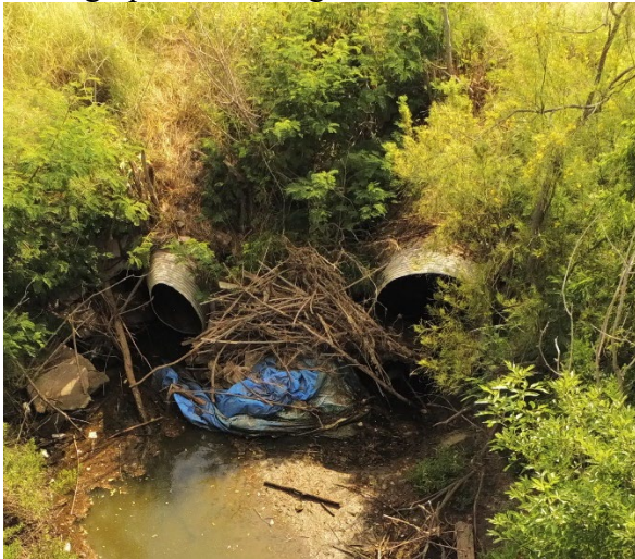
Photograph of upstream side this summer after a rain Note the collapsed end of the pipe on the left.
