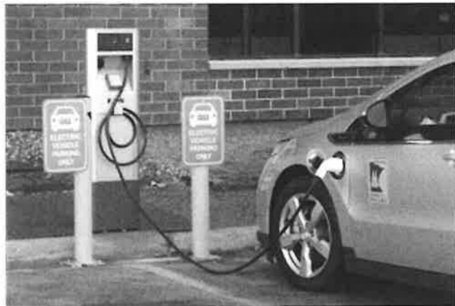
Example electric vehicle charging station
