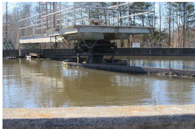
Figure 2.8 - In-service Clarifier
