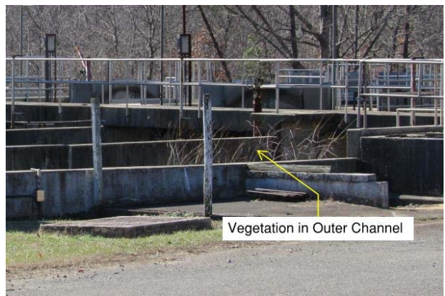
Figure 2.7 - Oxidation Ditch Outer Channel
