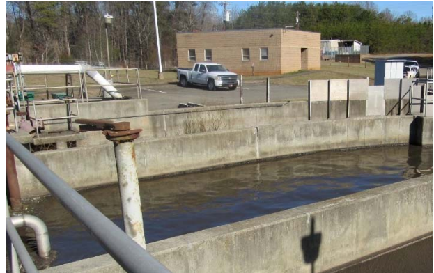
Figure 2.7 - Oxidation Ditch Outer Channel
