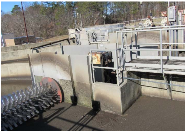
Figure 2.5 - Oxidation Ditch Piping
