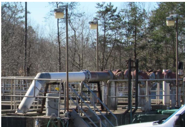
Figure 2.5 - Oxidation Ditch Piping
