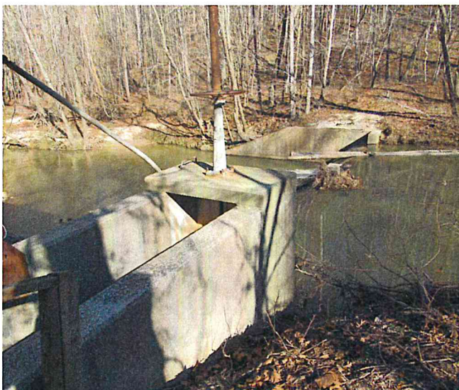
Pilot Mountain water treatment plant intake
