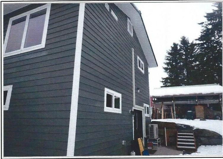
REAR OF SUBJECT PROPERTY
