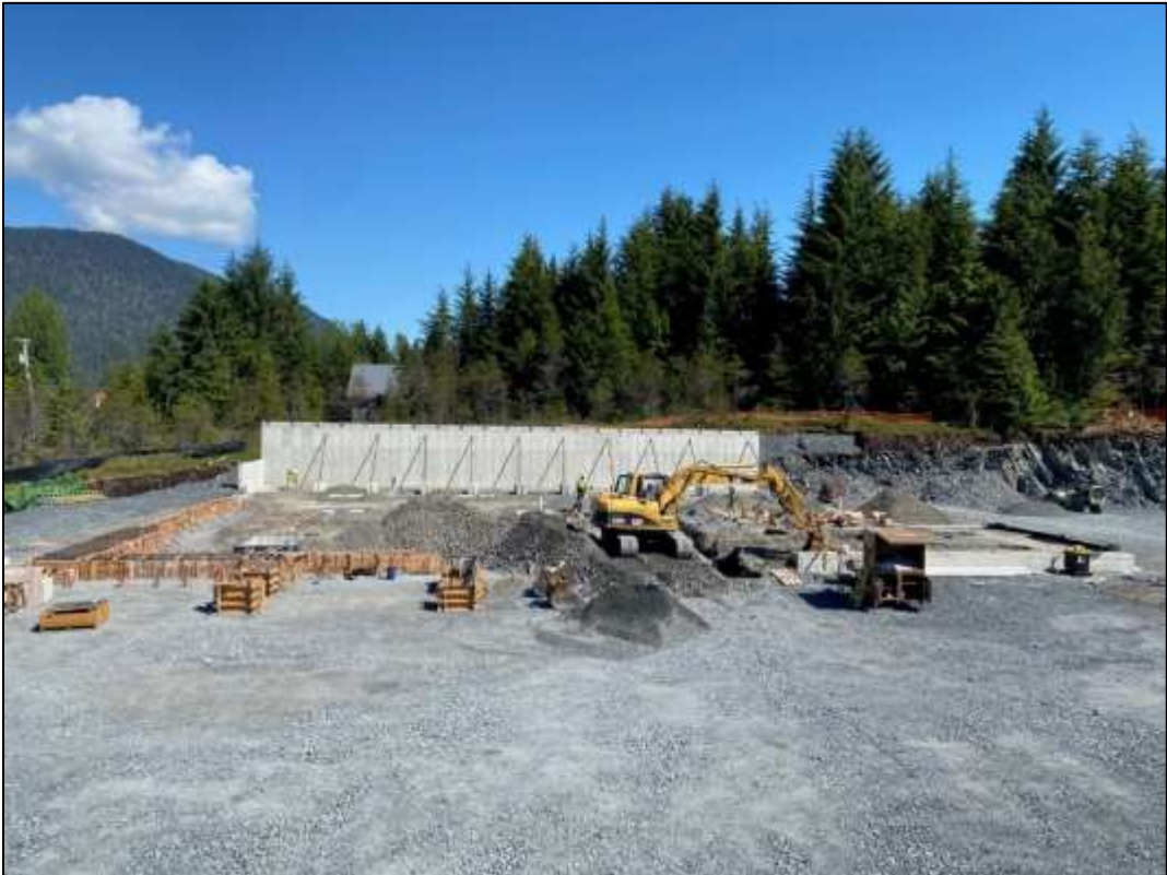
WERC Building Site 6/19/2024
