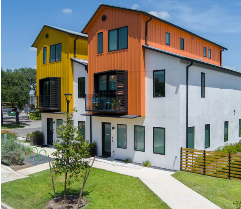
Compact, location-efficient housing in San Marcos, Texas (Credit: WGI)
