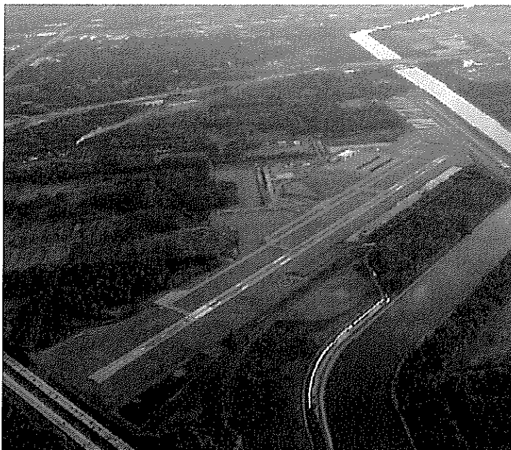
The FAA will consider releases from federal obligations, changes in use, and changes in designation according to the types of release requests in connection with the various federal obligations. In some cases, FAA's approval of a change in use is not a release of a specific federal obligation. Rather, it may represent FAA's concurrence with a sponsor's proposed change in use to eliminate any potential impact on a general federal obligation to provide aeronautical access and to operate and maintain infrastructure. For example, the FAA should not release property on the approach end of a runway if this results in a structure or construction that would impact the airport. As shown here, the highway on the lower left corner of the photograph has resulted in an extensive displaced threshold, diminishing the utility of the airport. (Photo: CAP)
