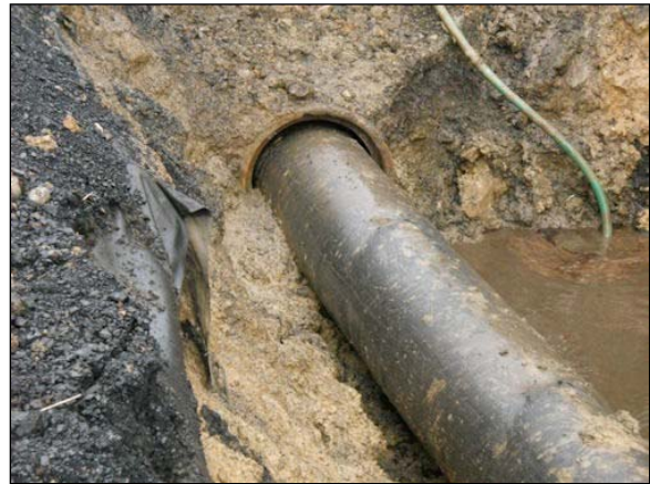
Figure 1: Sliplining with HDPE pipe
