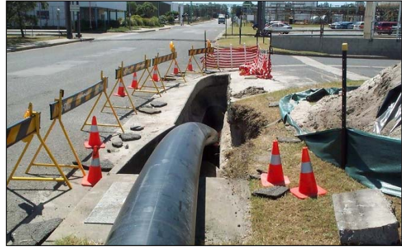
Figure 2: Insertion pit for sliplining with HDPE pipe
