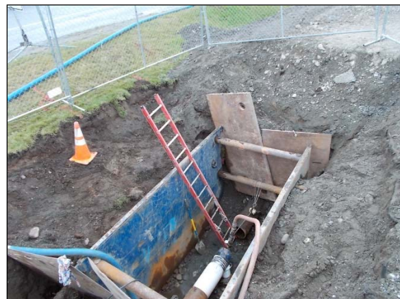
Figure 3: Typical CIPP liner access and insertion pit
