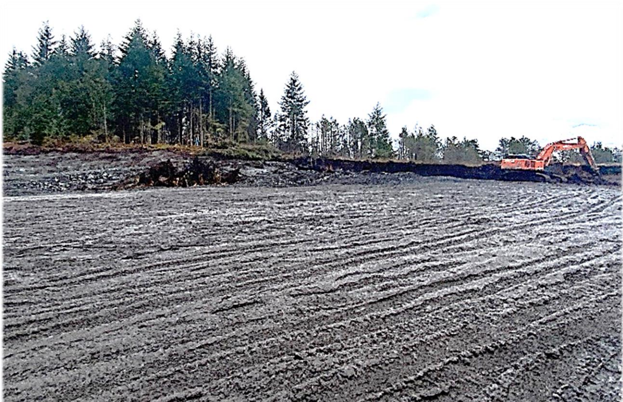
Main Hospital - LTC Building Site as of March 18th
