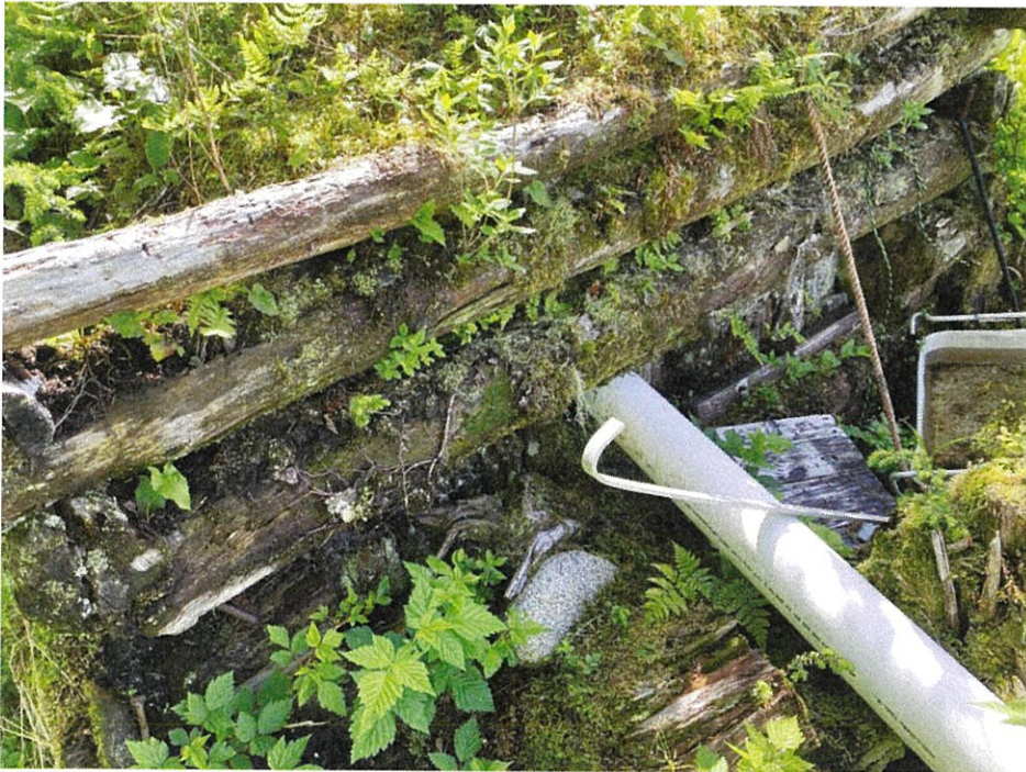
Pipe connected to septic tank and leading to beach.
