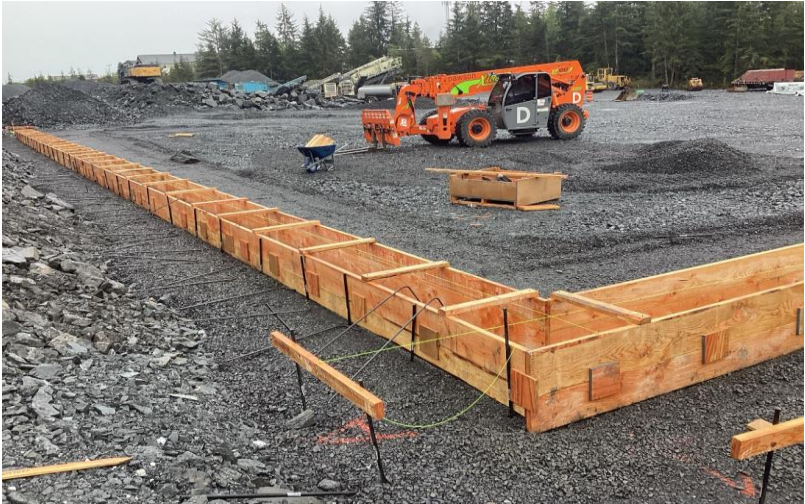
Footing Forms at Grid 1
