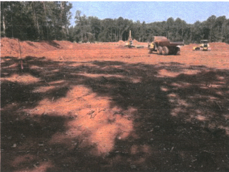
Lot 15 looking west
