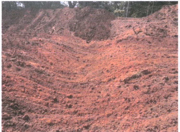
Existing ditch properly cleared out.
