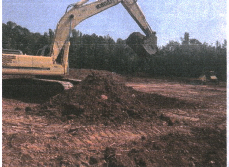
Remaining topsoil being removed while onsite.
