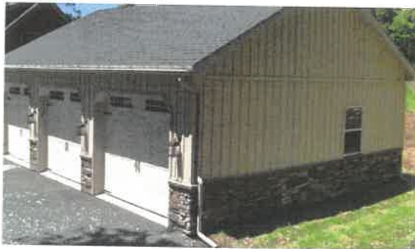
A similar example of the storage building style of stacked stone and metal siding.
