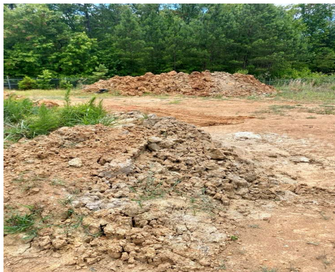
*Pictured above: Dried sludge being piled up for removal.
