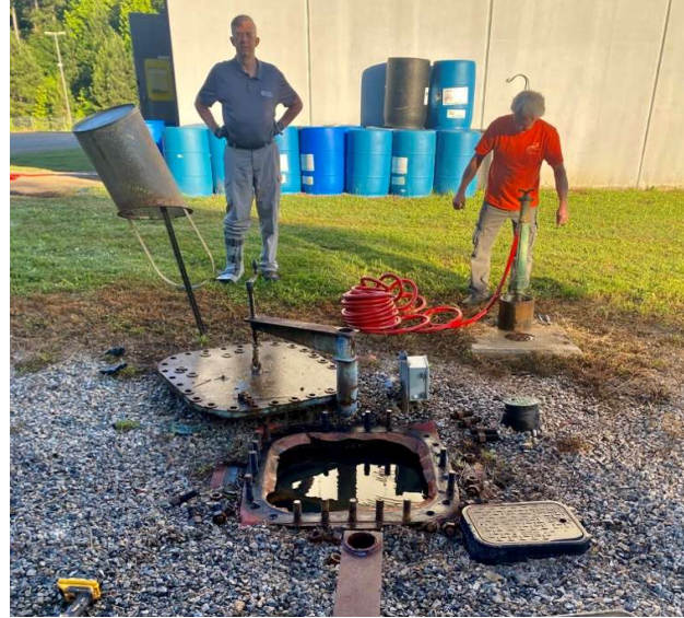
*Pictured above: left, cleaned basin; right, strainers being pulled and cleaned.
