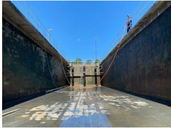
*Pictured left, almost 6 feet of sludge accumulated in less than 5 weeks due to the increased ambient air temperatures. Pictured right, cleaned sedimentation basin.
