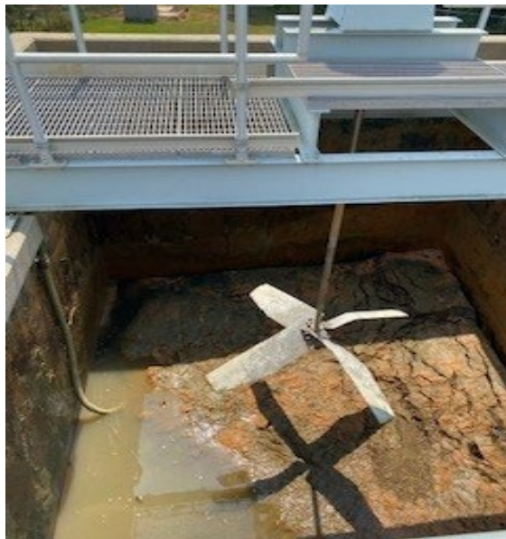
*Pictured left, before floc chamber cleaning. Pictured right, after floc chamber cleaning.
