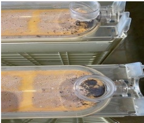
*Pictured left, manganese accumulation on the intake of the membrane cassette. This material is removed and strands are repaired.
