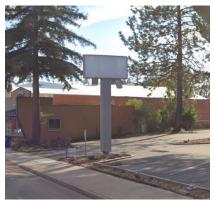
**Proposed Solution**: If the sign face is in good enough shape, flip the sign face around (inverted graphics may be slightly visible) being sure to verify any illuminated signs are powered down.
