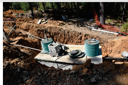
Septic Tank & STEP pipe
