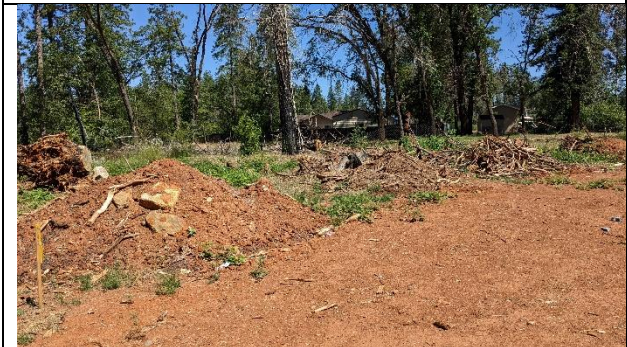
Photo 7. Ground clearing activity looking east.
