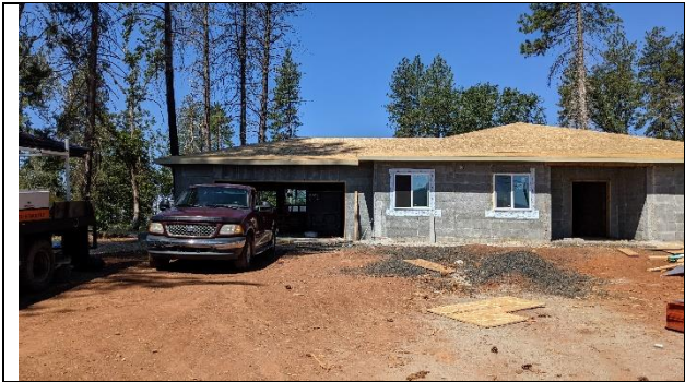
Photo 1. House 1 looking west.
