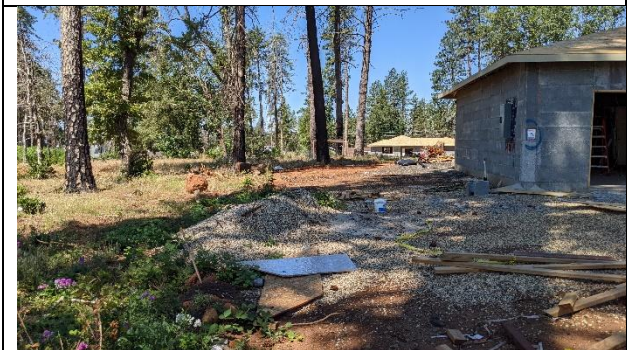
Photo 3. General project area looking west.
