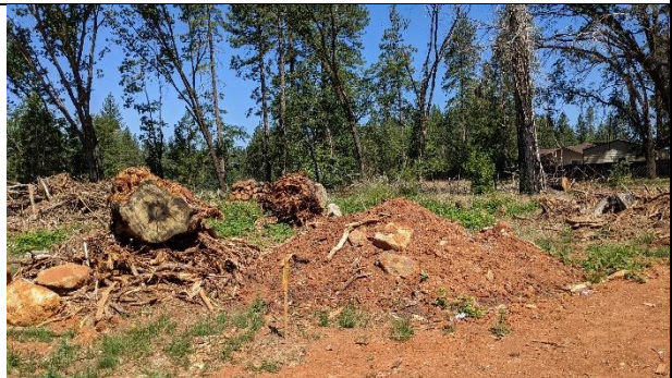
Photo 8. Ground clearing activity looking east.
