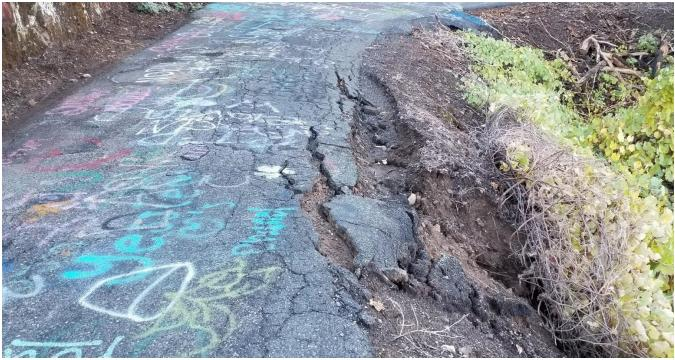
Honey Run Road – Graffiti and pavement failure along downhill edge
