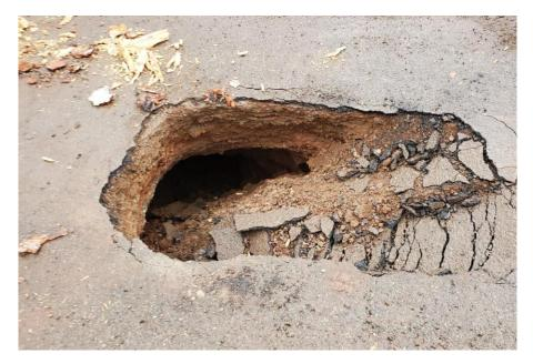
Figure 1 - Stearns Road Void Caused by Erosion
