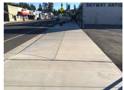
Example of new sidewalk with driveway conforms
