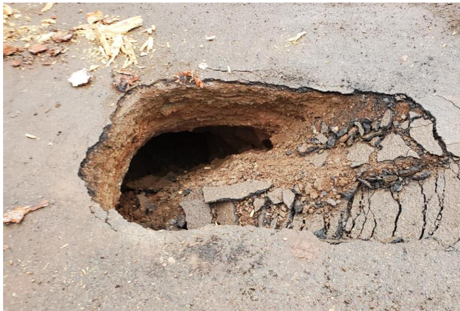
Figure 1 - Stearns Road Void Caused by Erosion
