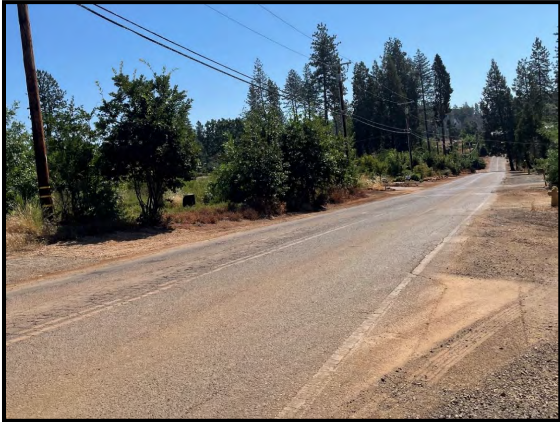
Central Park Dr. Speed Survey Location
