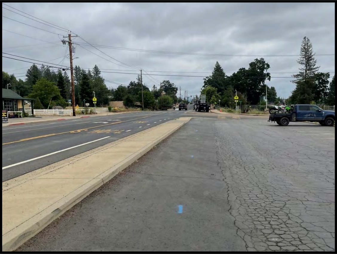
Pearson Rd. Speed Survey Location
