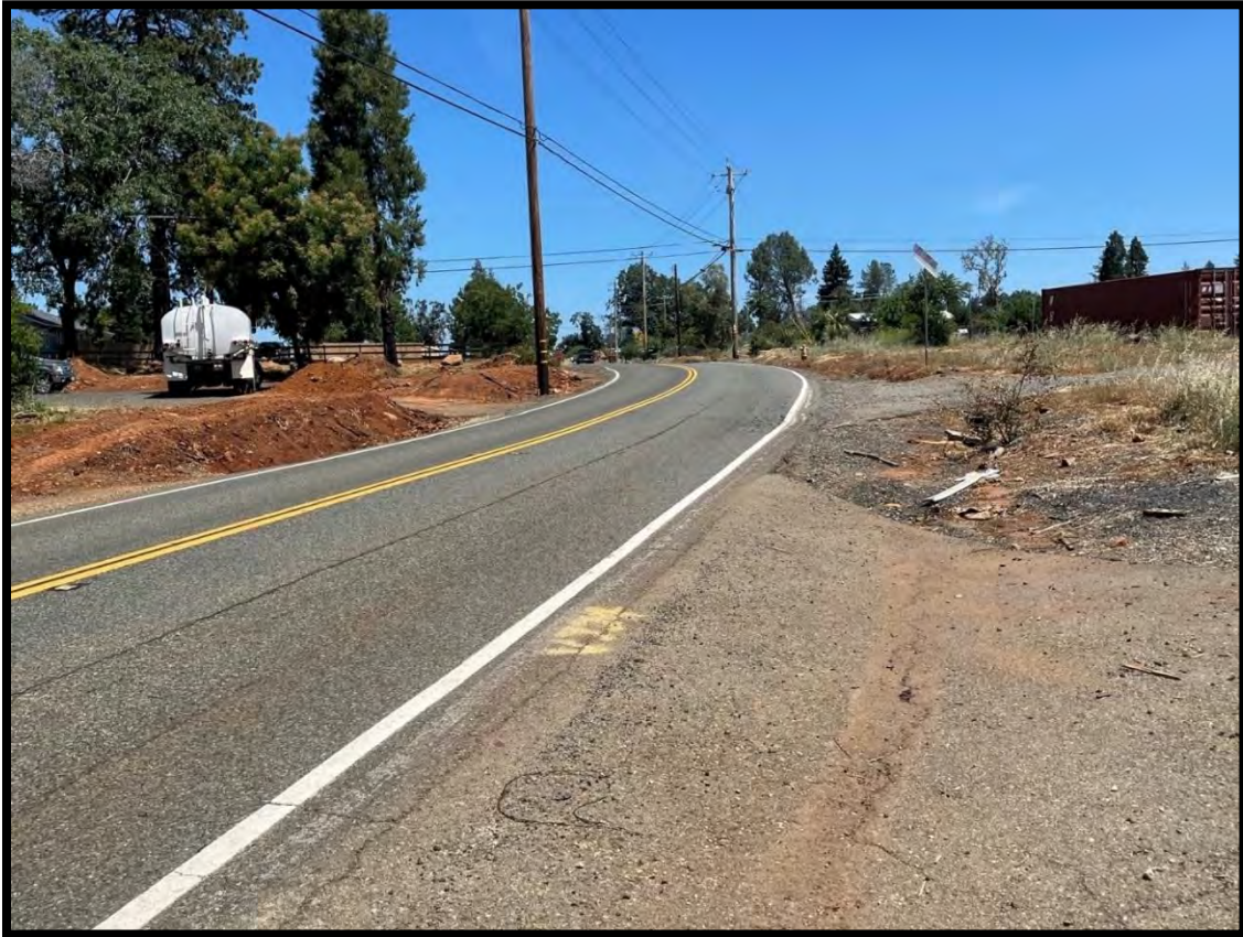
Neal Rd. Speed Survey Location
