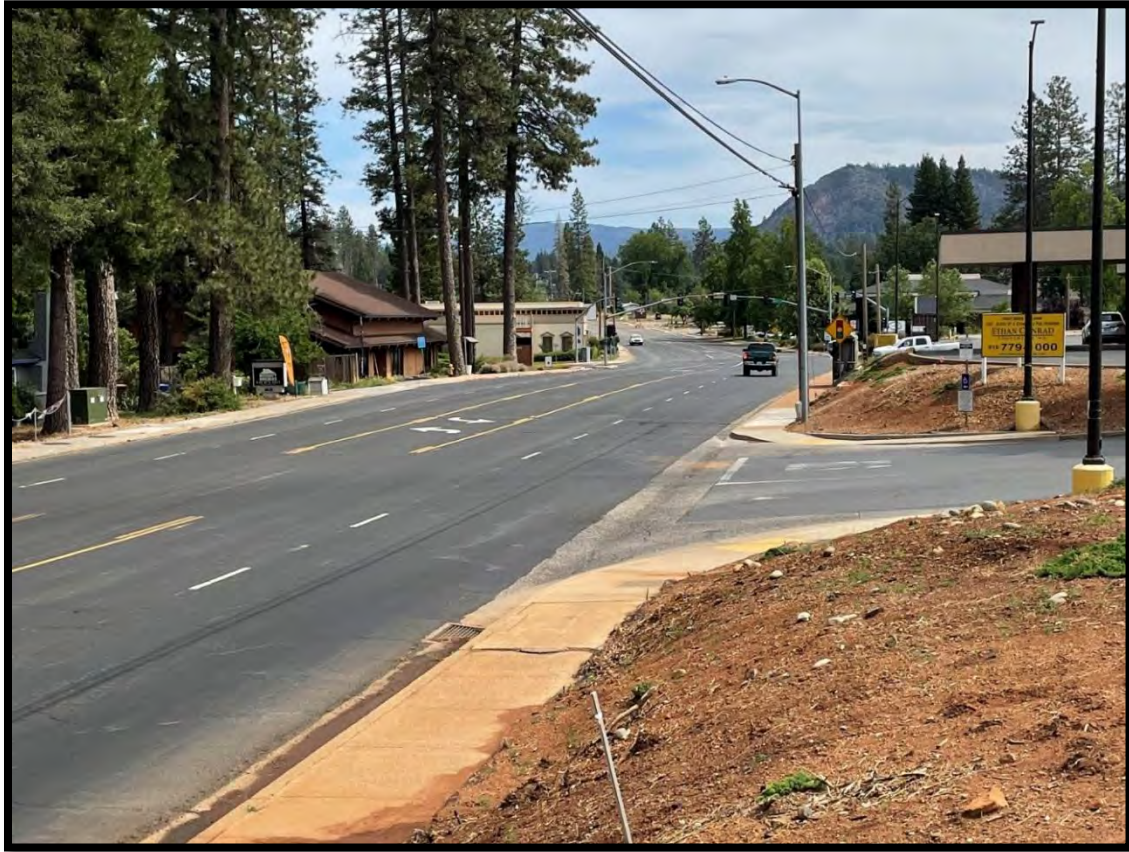
Clark Rd. Speed Survey Location
