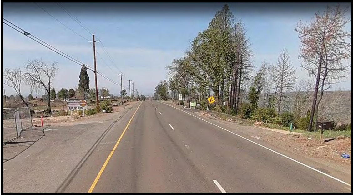
Skyway (WB) Speed Survey Location
