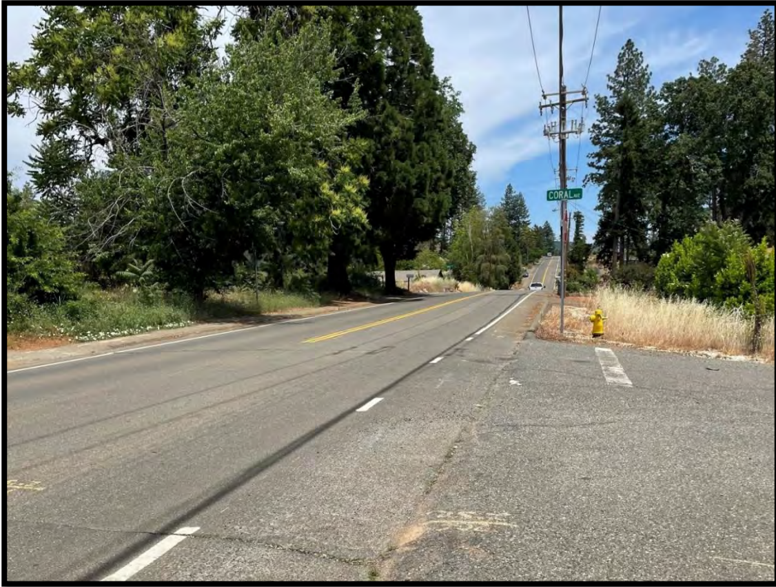
Bille Rd. Speed Survey Location
