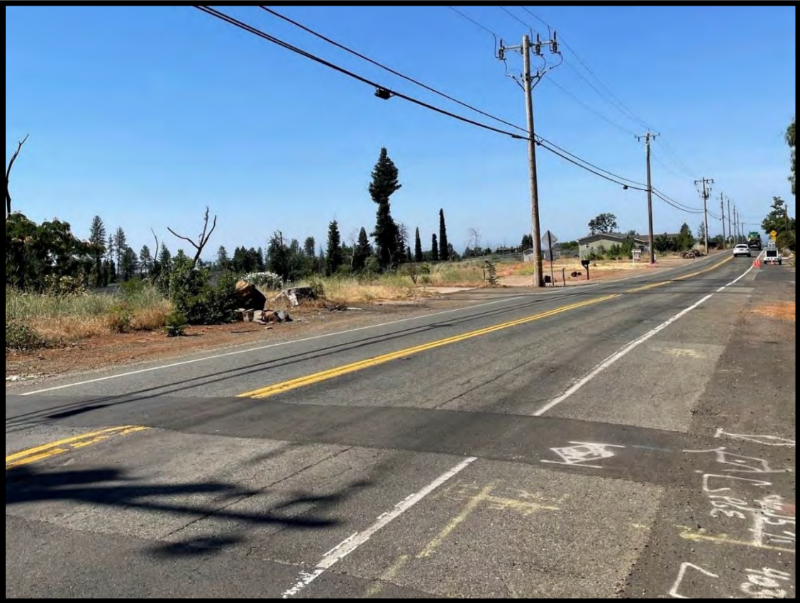
Neal Rd. Speed Survey Location
