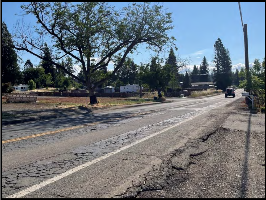
Bille Rd. Speed Survey Location
