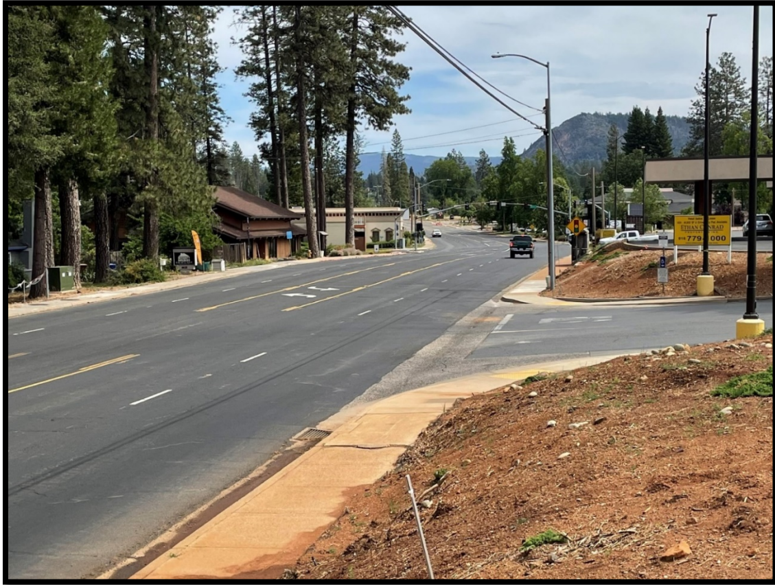
Clark Rd. Speed Survey Location
