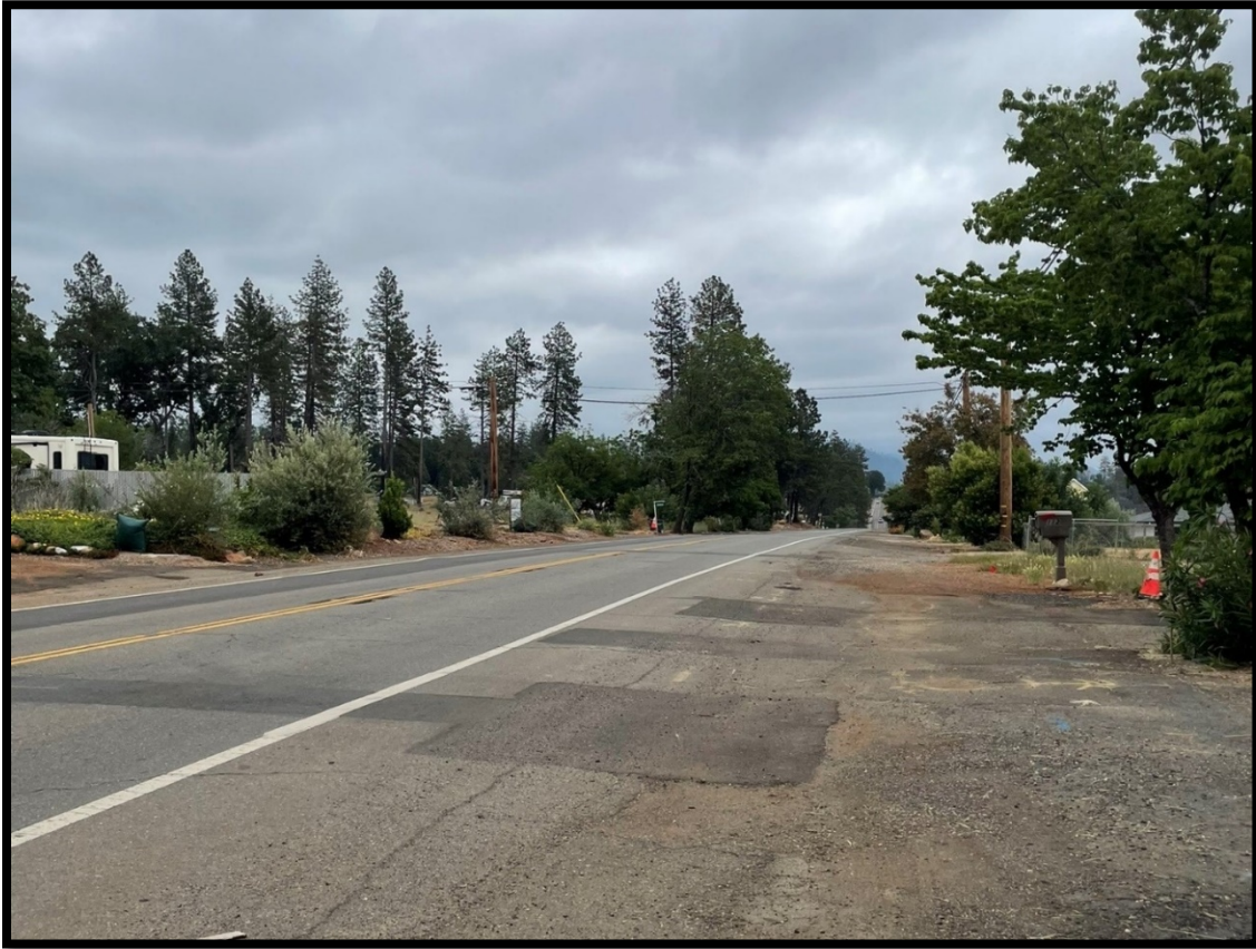
Pearson Rd. Speed Survey Location
