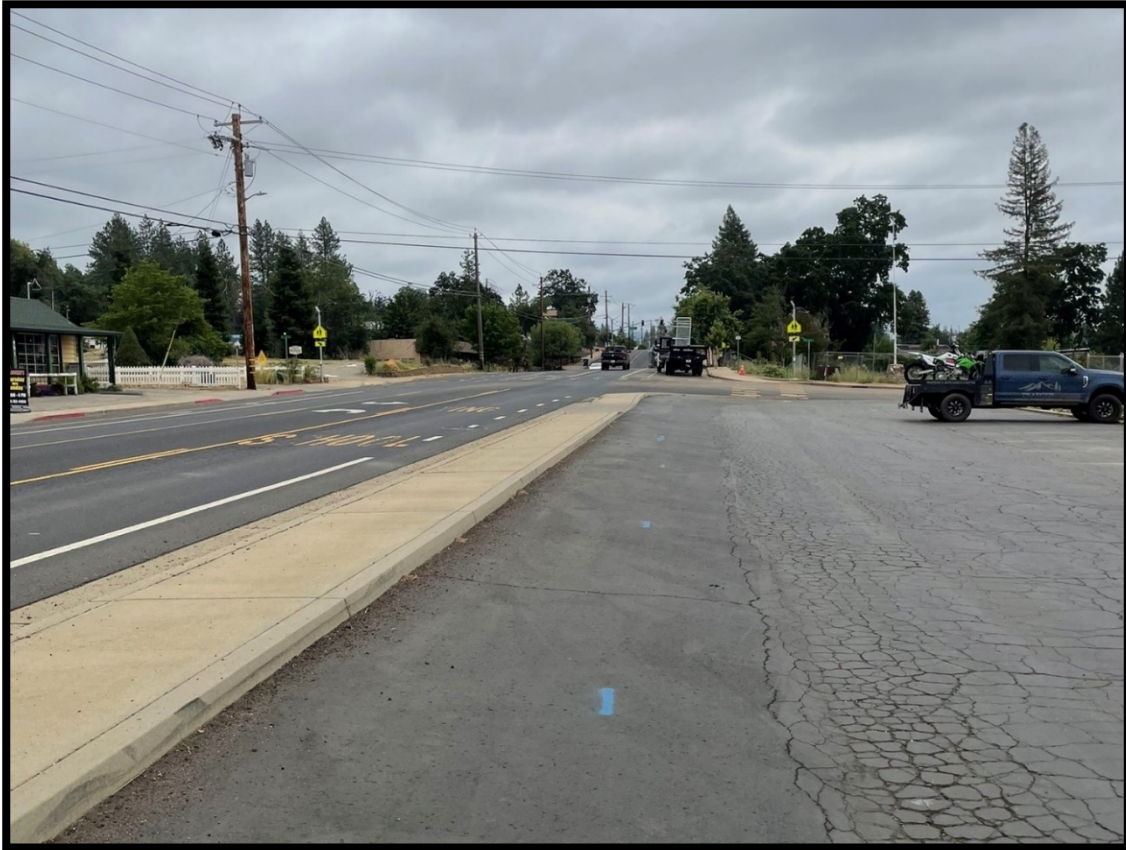
Pearson Rd. Speed Survey Location
