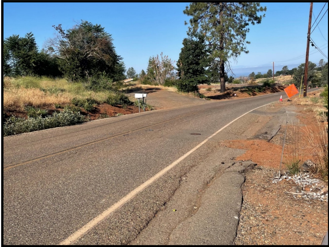
Honey Run Rd. Speed Survey Location
