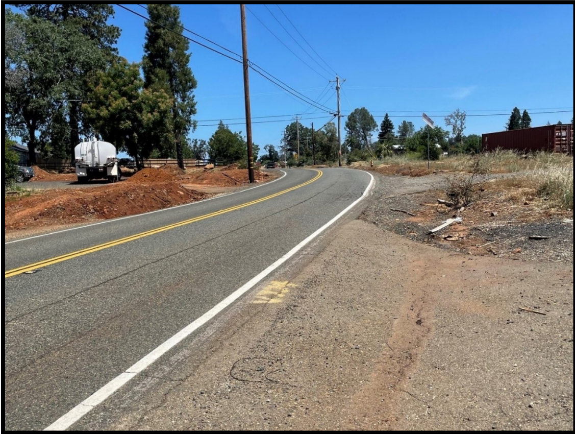
Neal Rd. Speed Survey Location
