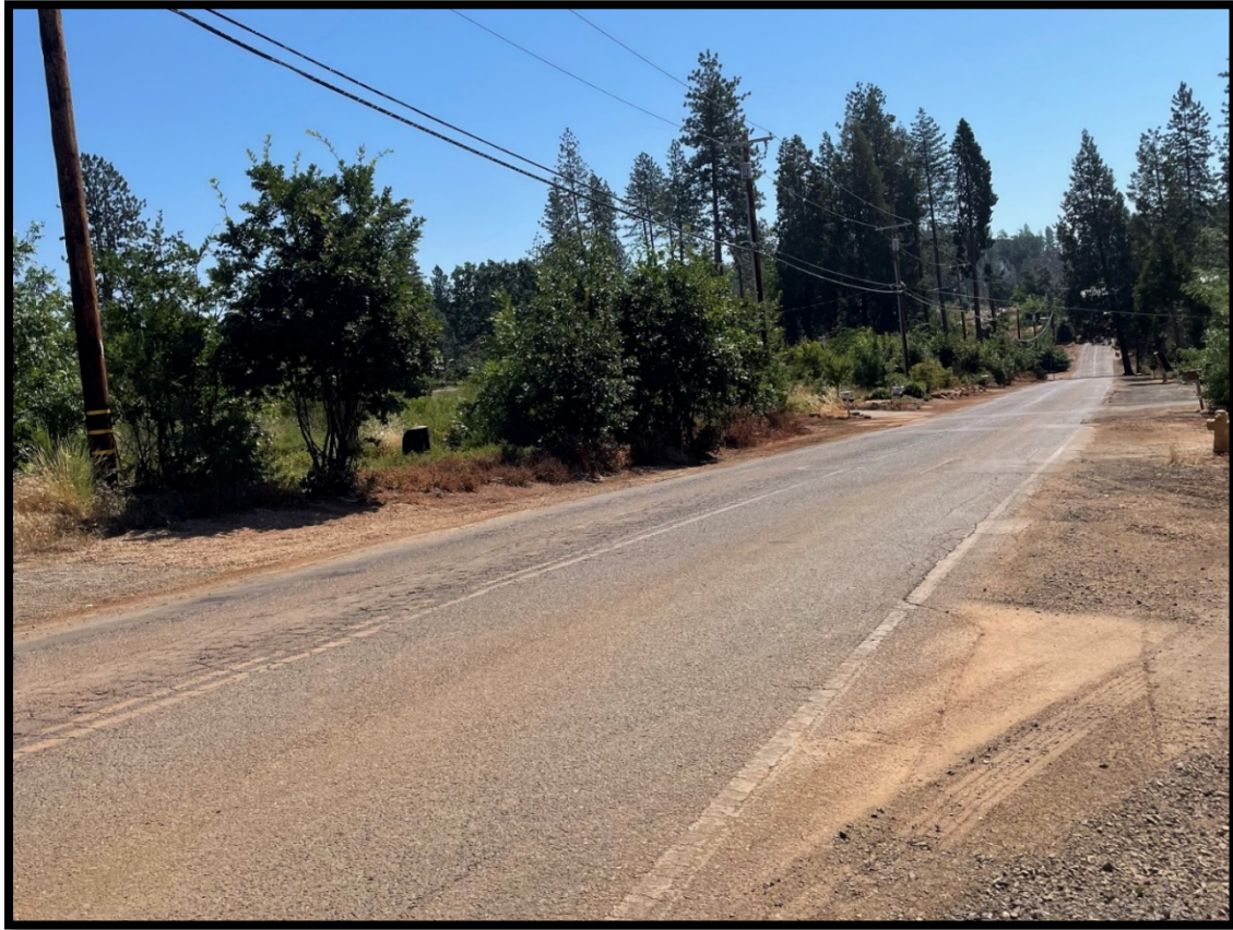
Central Park Dr. Speed Survey Location
