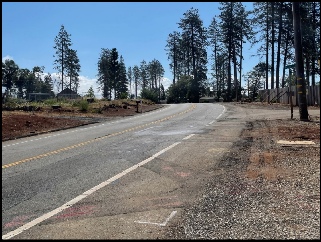
Pearson Rd. Speed Survey Location
