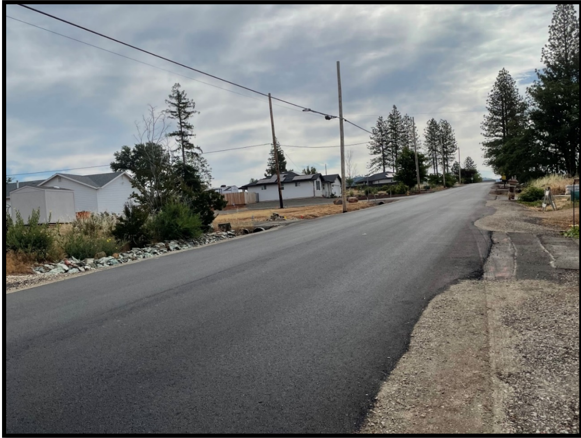
Stearns Rd. Speed Survey Location
