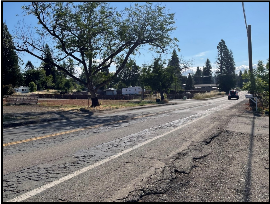
Bille Rd. Speed Survey Location
