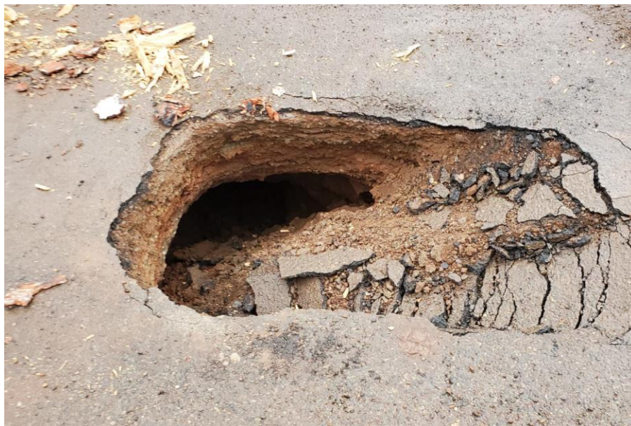
Figure 1 - Stearns Road Void Caused by Erosion Upon Discovery
