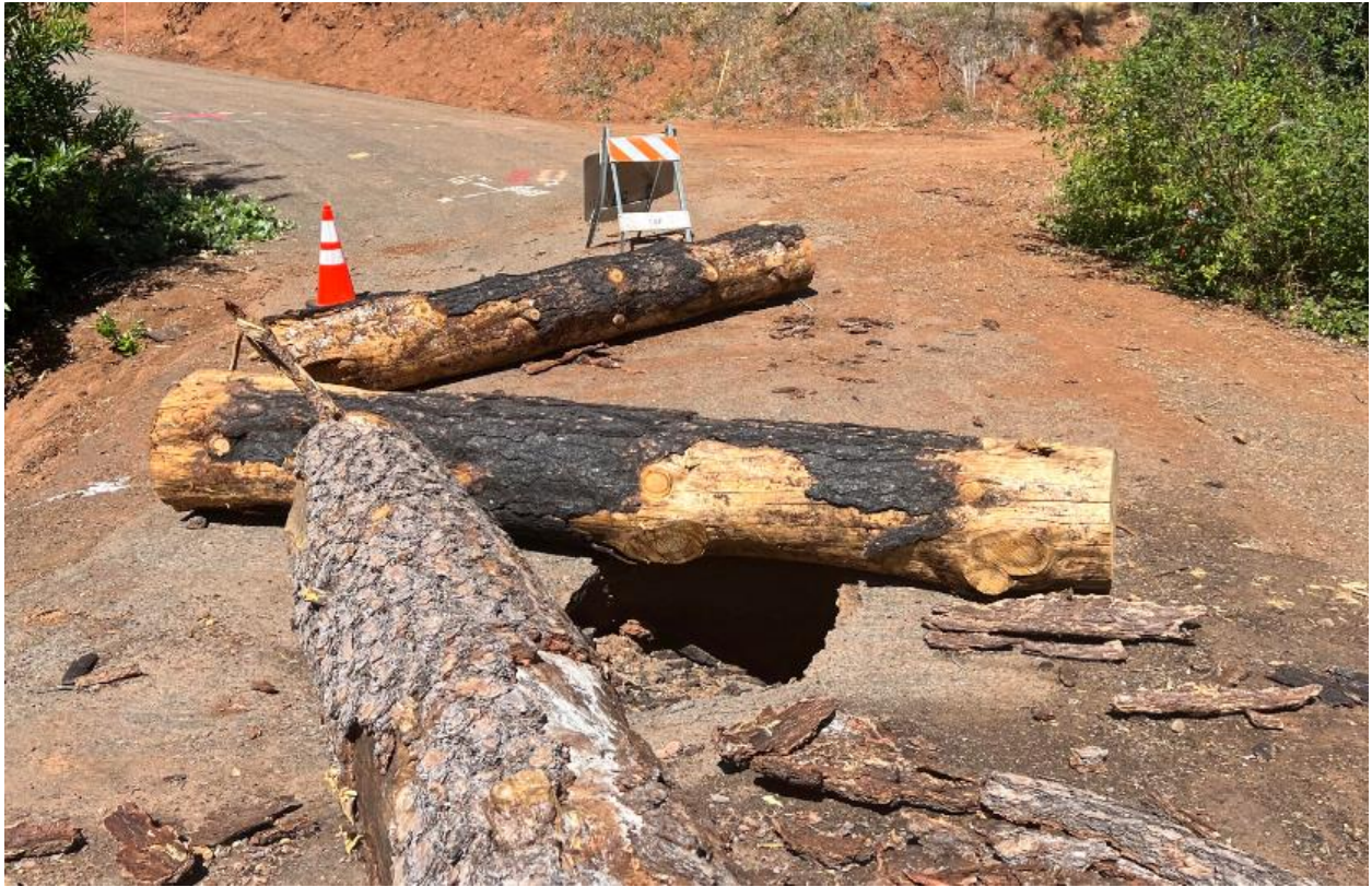
Figure 2 - Stearns Road Void Existing Condition (Logs for Closure)
