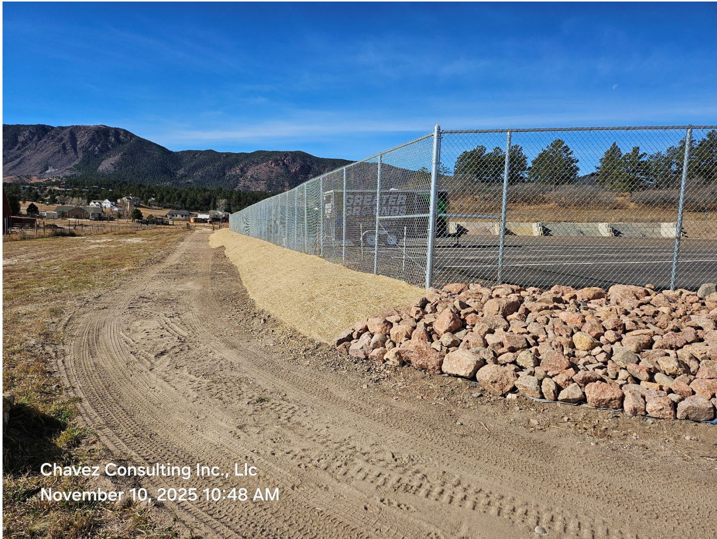
Figure 6. Greater Grounds (south property line): erosion control blanket installed.
