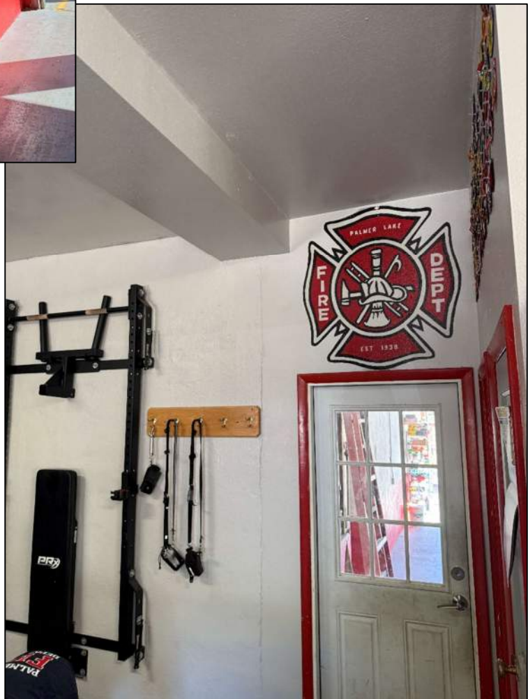
Photo 10: Beam and bearing location inside bunkhouse looking east.
