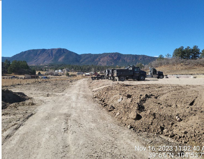
Figure 1. Northeast property corner, looking south down east property line. No stormwater control measures in use.
