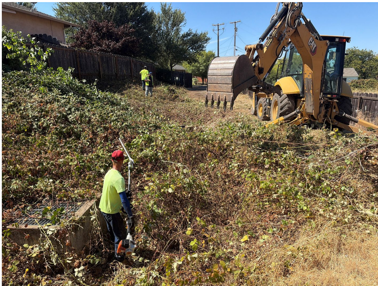
ABATEMENT OF VEGETATION CITY OWNED PROPERTY NEAR CAL WATER HEADQUARTERS
