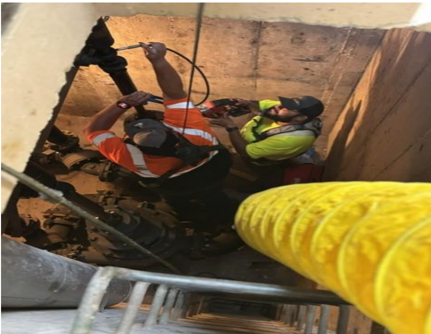
Greased the centrifugal pumps at Olive Glen lift station.
