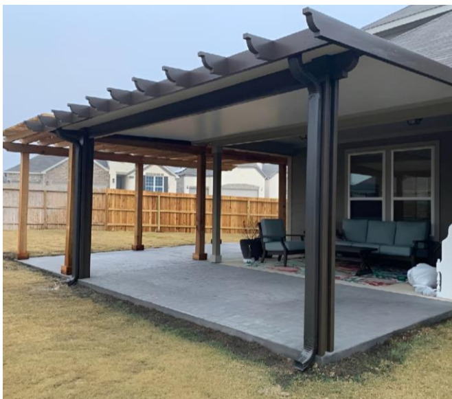
IMAGE 3 – Accessory Structure, Patio Cover
