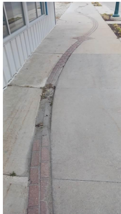
Paver band setting greater than 0.25
