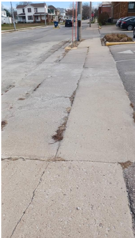
Panel displacement
