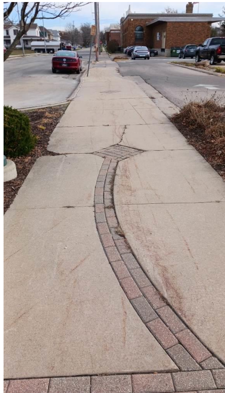
Paver and diamond settling
