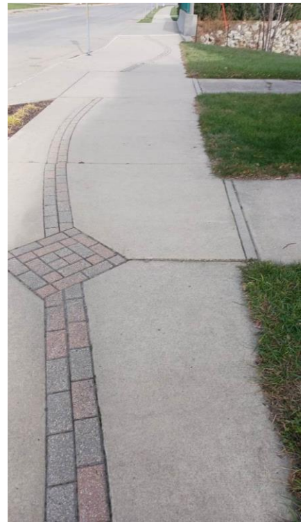
PCC displacement across paver band
