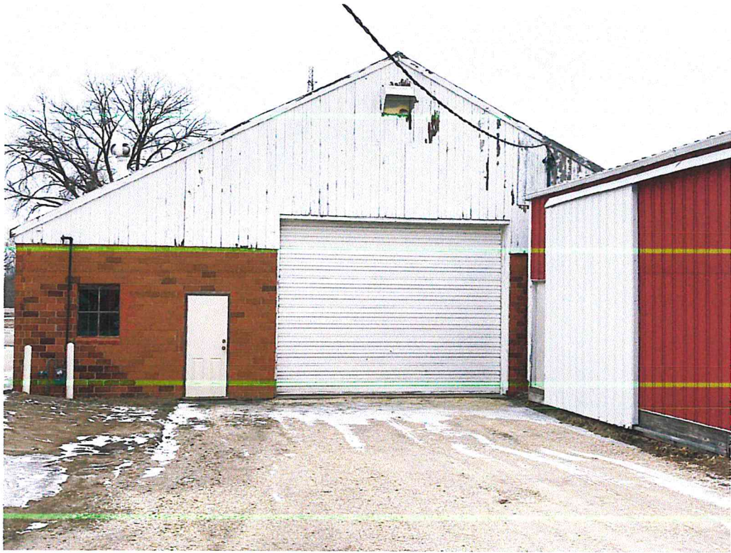
View of back of building.
