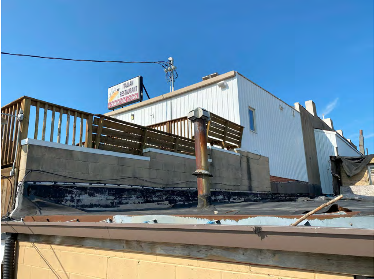
Southeast wall/parapet-wall showing deck buildout
