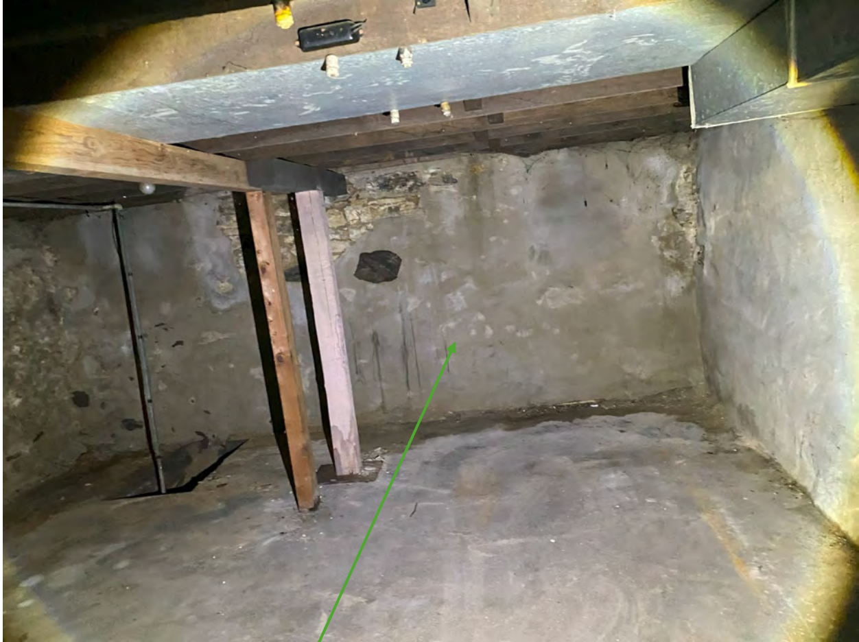
West foundation wall
