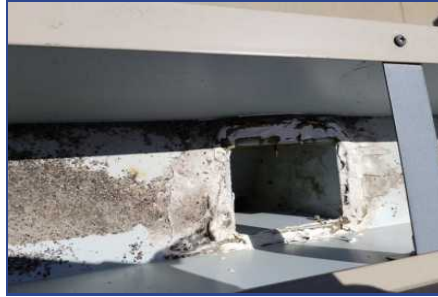
Section A - Deficiency #6 Failing sealant
