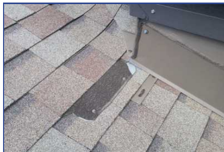
Section B - Deficiency #5 Poorly installed flashing
