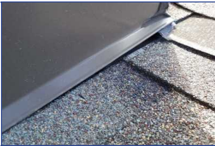
Section B - Deficiency #6 Curb improperly slashed
