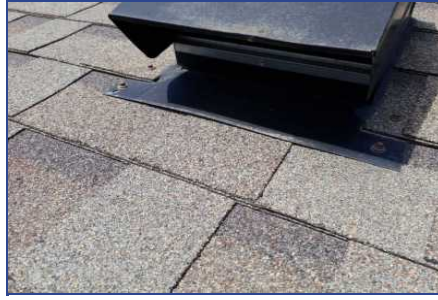
Section A - Deficiency #5 Heavily rusted kitchen exhaust vent
