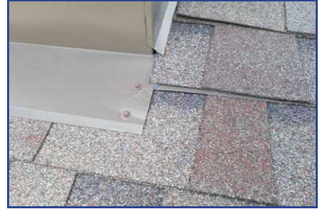
Section B - Deficiency #5 Poorly installed flashing
