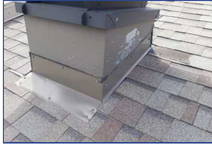
Section B - Deficiency #5 Poorly installed flashing
