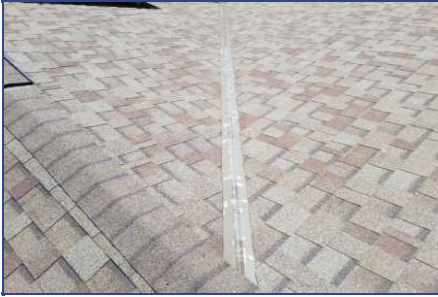
Section B - Deficiency #3 Deteriorated valley tin
