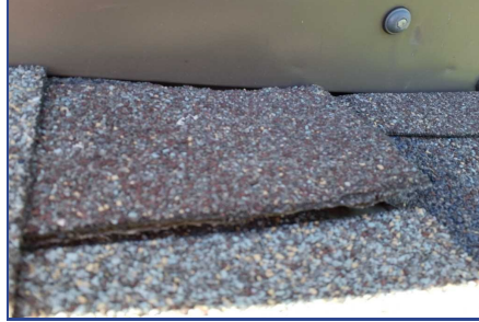
Section A - Deficiency #2 Improperly flashed pillars
