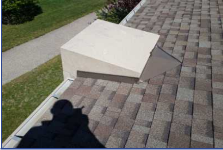
Section A - Deficiency #2 Improperly flashed pillars
