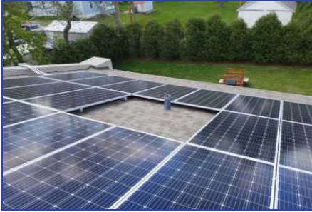
Section B - Deficiency #4 Improper Plumbing pipe flashing
