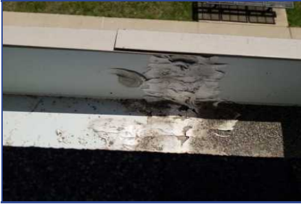
Section A - Deficiency #6 Failing sealant
