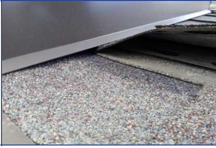
Section B - Deficiency #5 Poorly installed flashing
