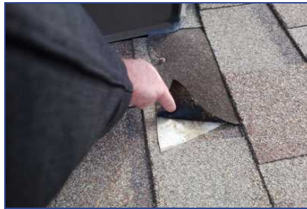
Section B - Deficiency #5 Poorly installed flashing
