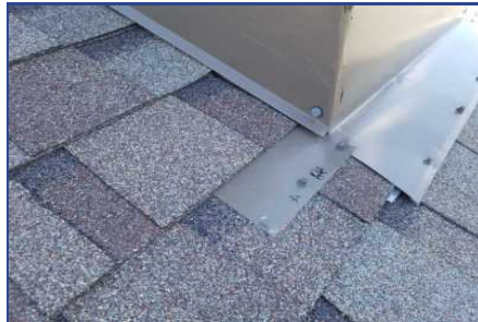
Section A - Deficiency #3 Improperly flashed in roof vent
