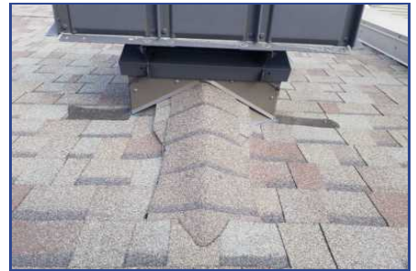
Section B - Deficiency #5 Poorly installed flashing
