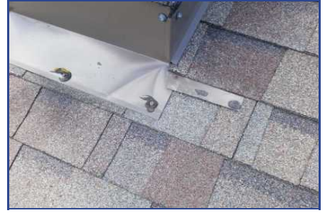
Section B - Deficiency #6 Curb improperly slashed
