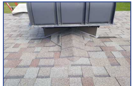
Section B - Deficiency #5 Poorly installed flashing
