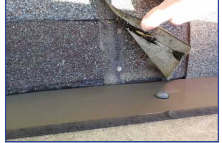
Section A - Deficiency #2 Improperly flashed pillars
