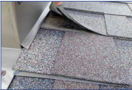
Section B - Deficiency #5 Poorly installed flashing
