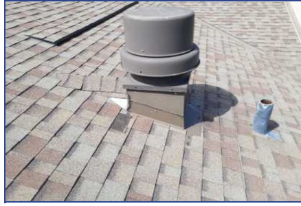
Section B - Deficiency #6 Curb improperly slashed
