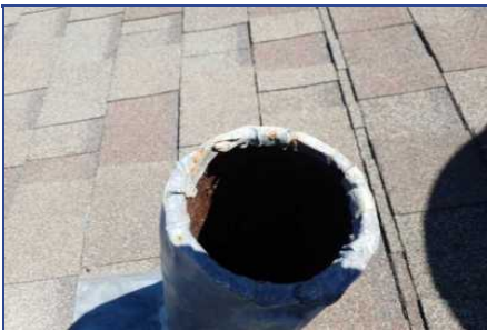
Section B - Deficiency #1 Rusted Lead Top
