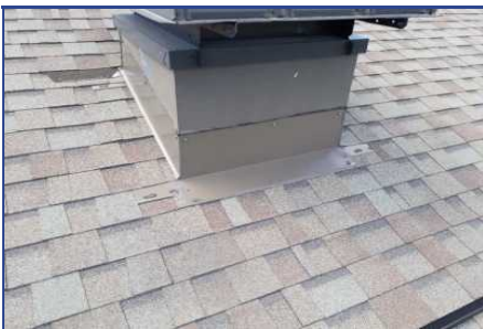
Section B - Deficiency #5 Poorly installed flashing
