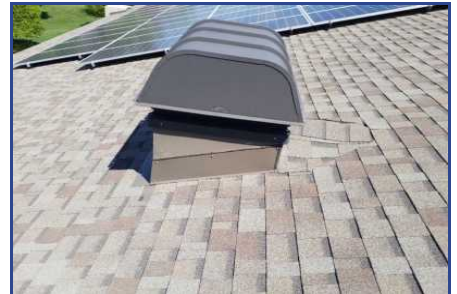
Section A - Deficiency #3 Improperly flashed in roof vent
