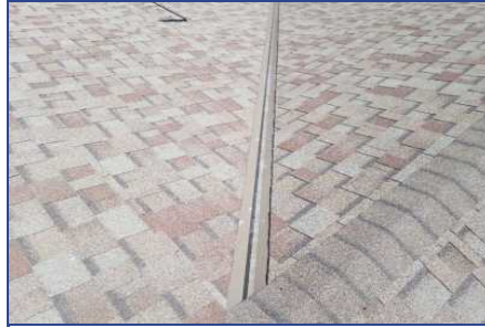
Section B - Deficiency #3 Deteriorated valley tin
