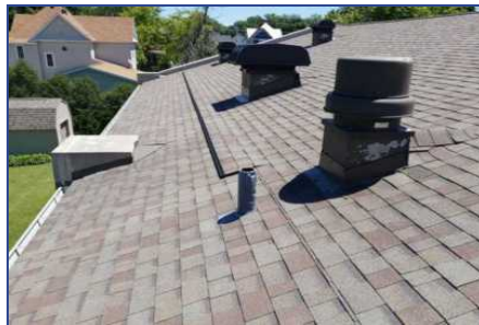
Section B - Deficiency #1 Rusted Lead Top
