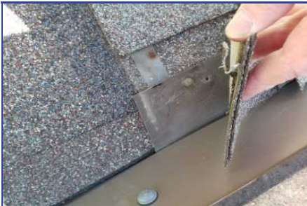
Section A - Deficiency #2 Improperly flashed pillars
