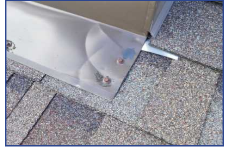
Section B - Deficiency #6 Curb improperly slashed
