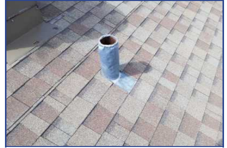
Section B - Deficiency #4 Improper Plumbing pipe flashing
