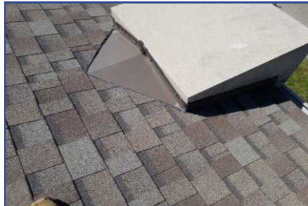
Section A - Deficiency #2 Improperly flashed pillars
