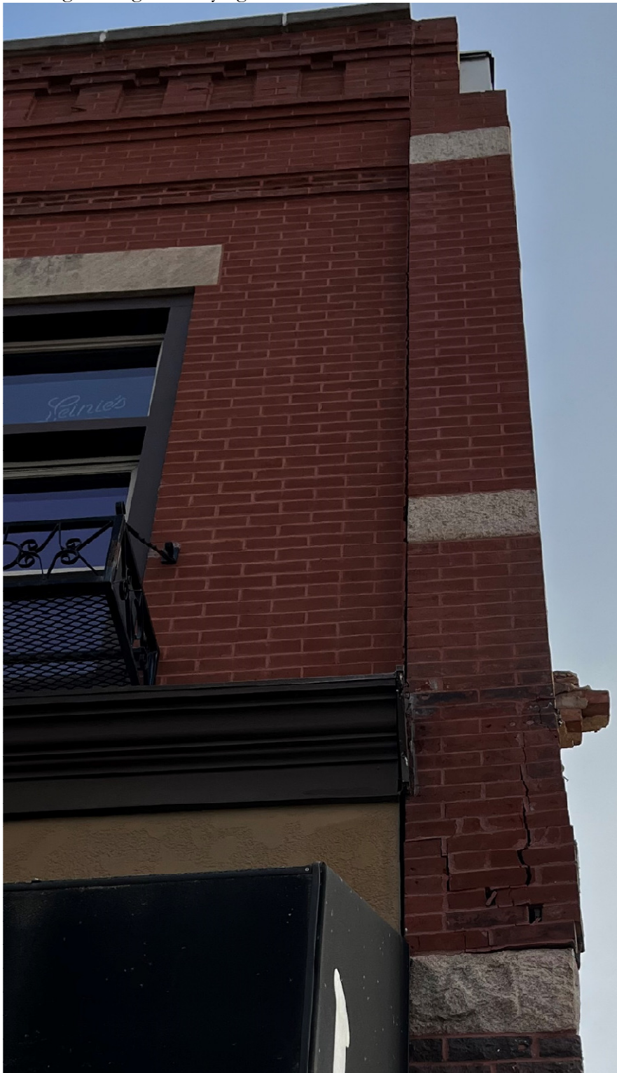
Figure 2: Opening in joint after demolition
