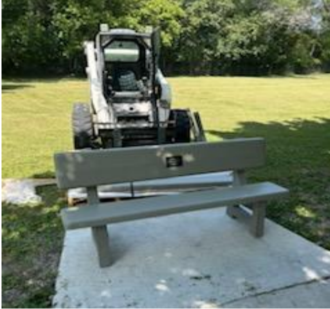
MEMORIAL BENCH INSTALLED
